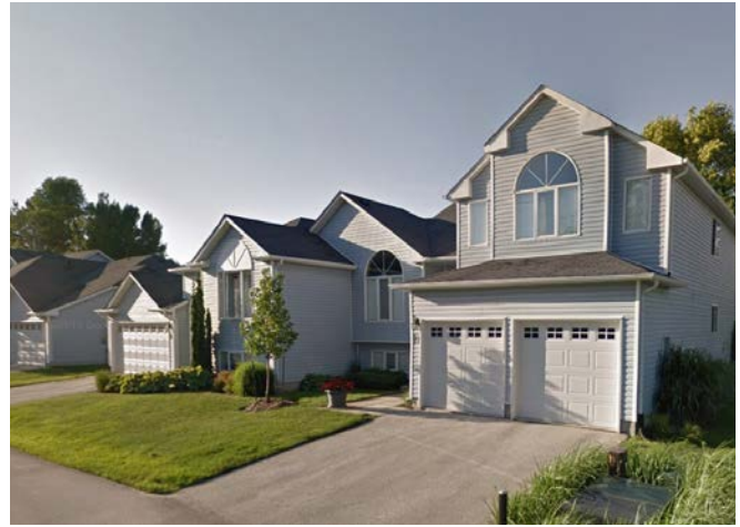
Existing built form on Sundial Ct east of the site
