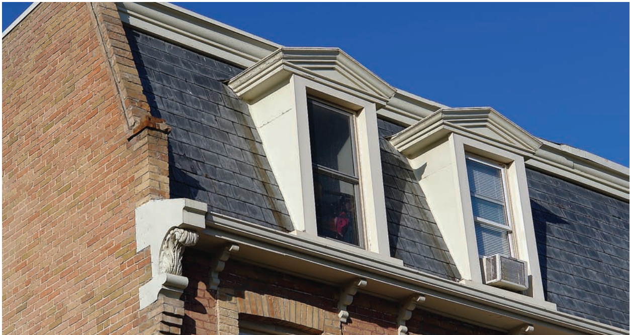
Mansard Roof, Ste. Marie Street
