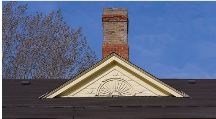
Roof Detail, 36 Ste. Marie Street
