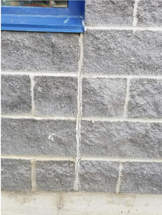
**Figure 33 Main Plant Building – Exterior - Masonry Control Joints**
