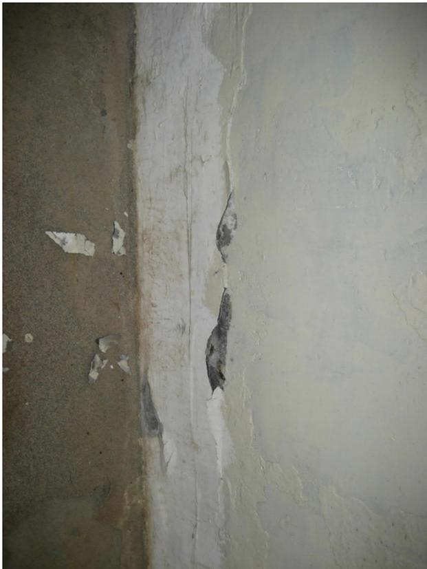
**Figure 53 Main Plant Building – Membrane Room - Wall Spalling**
