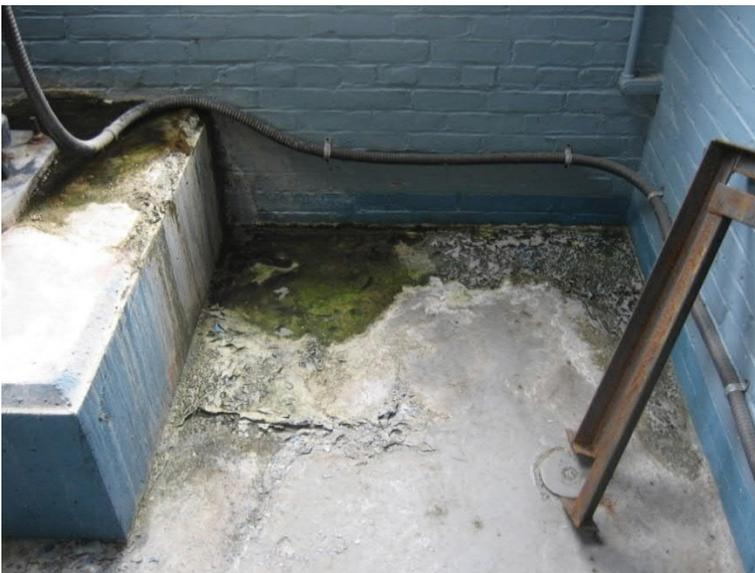
**Figure 12 Industrial Building - Deteriorated Ground Floor**
