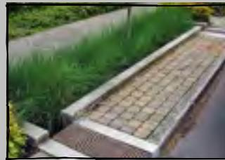
Decorative design for functional elements such as this curb, planter and grate for a stormwater rain garden, can be integrated into a site to create a unique character.
