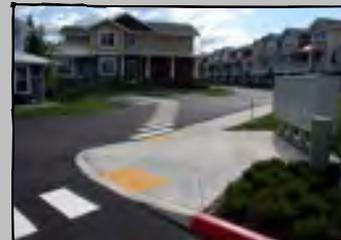
Example of truncated domes used at a pedestrian crossing to indicate transition from the sidewalk into the street crossing.
