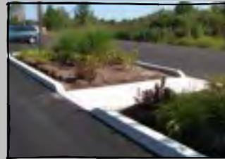
Pictured is an example of a walkway design that allows stormwater to enter a planter area as part of a Low Impact Development stormwater management system.
