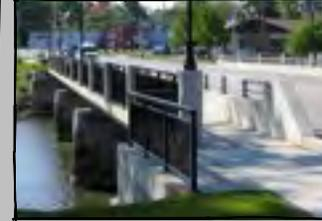
This large multiple lane bridge is designed with a dedicated pedestrian walkway that is physically separated from traffic as per the UDM requirements. Source: Dan Burden
