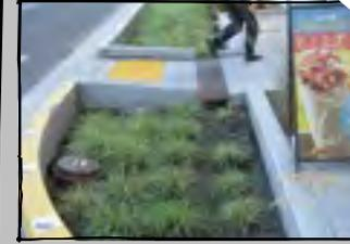
Example of LID stormwater management that includes bio-retention in the planter strip next to the sidewalk.
