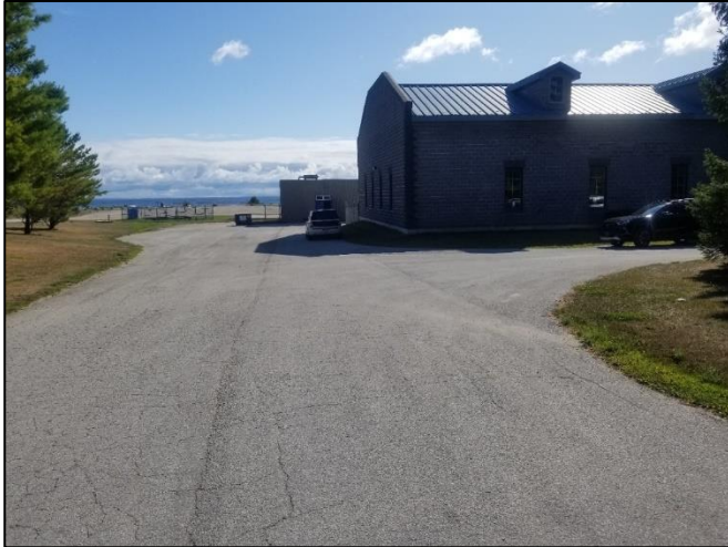
Photo 5: Visually confirmed disturbance (building footprint, access road construction), facing east
