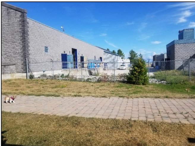
Photo 9: Visually confirmed disturbance, building footprint and infrastructure), facing north
