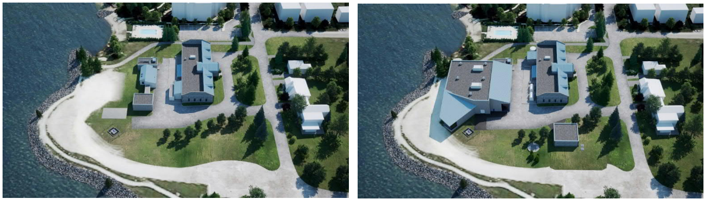
Figure 34 North Aerial View of the Existing Infrastructure and Optional Concept to Achieve Ultimate Flows
