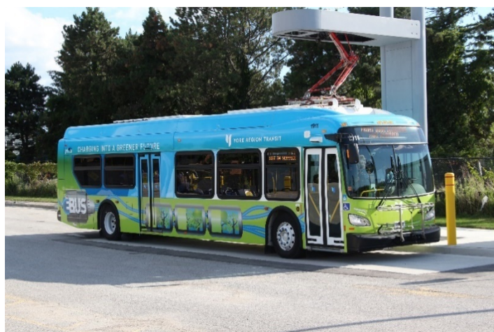
Exhibit 8-2: In-Service BEB Charging System, York Region Transit
