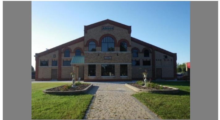
Street level access with clear path of travel at the Curling Club.
